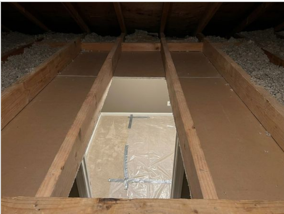
Attic — ceiling opening into Bedroom 3 after removal of the affected board
