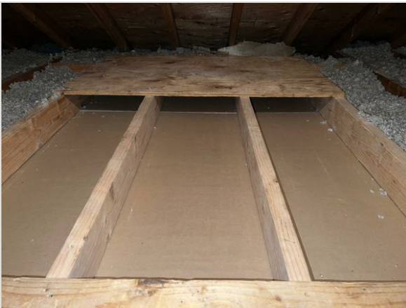
Attic — ceiling joist bays stripped of insulation and cleaned
