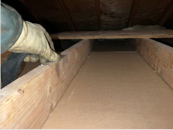
Attic — surface tape lift S-306 on the cleaned ceiling joist and platform decking
