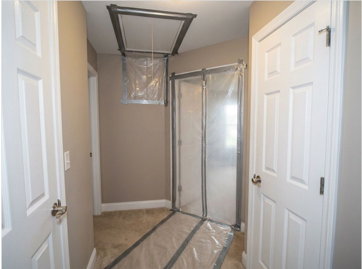
Upstairs hallway showing the polyethylene containment barrier sealing the Bedroom 3 doorway, with secondary poly covering over the ceiling register overhead. Floor protected with poly sheeting. No mold growth, water staining, or active moisture damage visible.
