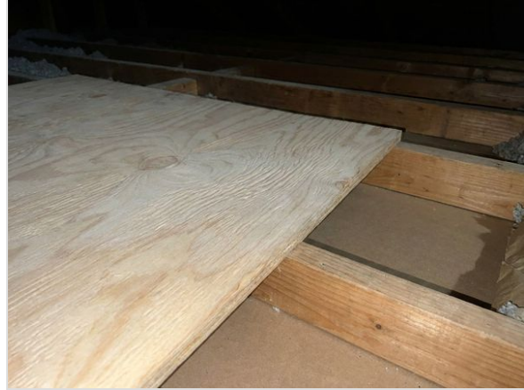
Attic — platform decking after HEPA vacuuming and damp wiping
