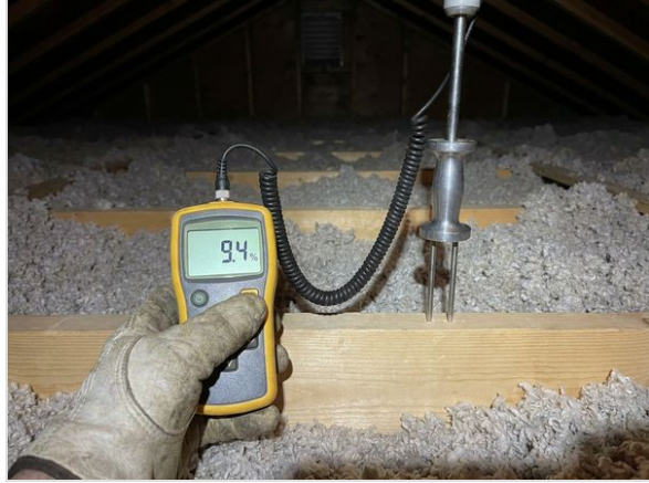
Attic — north gable rafter tie, re-established as the project dry standard
