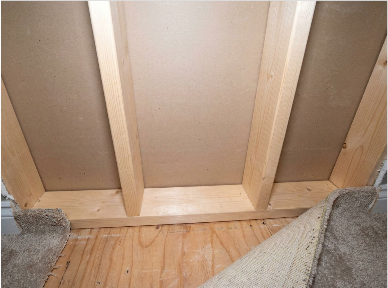
Low-angle view of the west wall base showing exposed SPF framing, bottom plate, and OSB subfloor after carpet and pad removal. No visible mold growth, staining, or moisture damage on any surface in frame.
